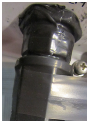
Figure 3.6. Wrapping the Connector with Rubber-splicing or Self-amalgamating Tape
